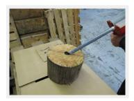
8. Using continuous motion, proceed dispensing to the outer circumference of the pole depositing even beads in a circular motion toward the center starting point.
